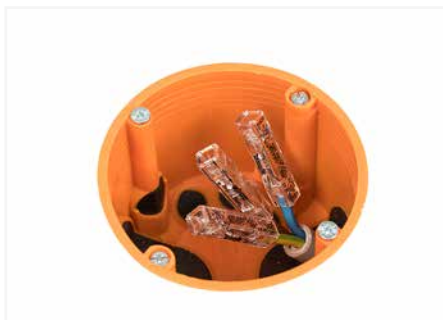
Extending short wires.
