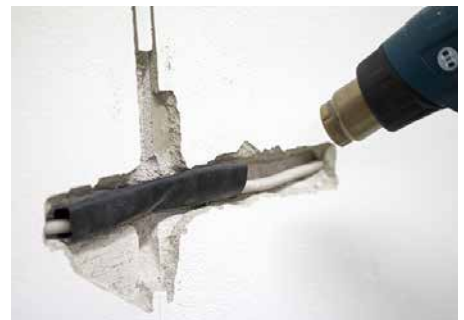
Heat the shrink tube and properly reclose the damaged area.
